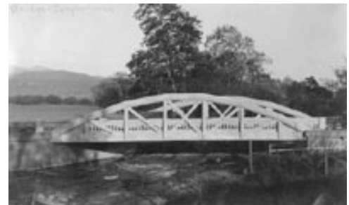
Highway Bridge Over the Creek (Carpinteria Valley Historical Museum).
