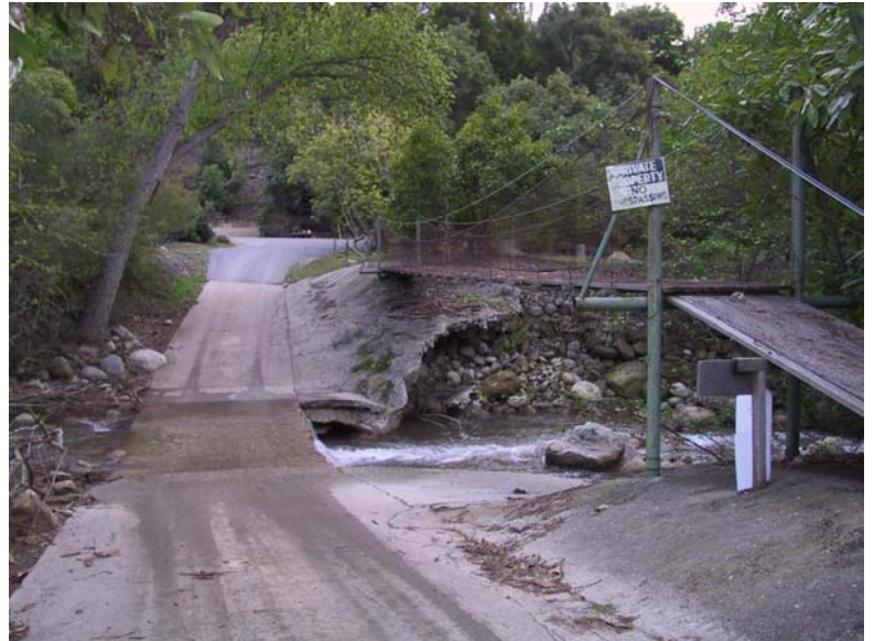
Upstream barrier, BR_CA_GR_4
